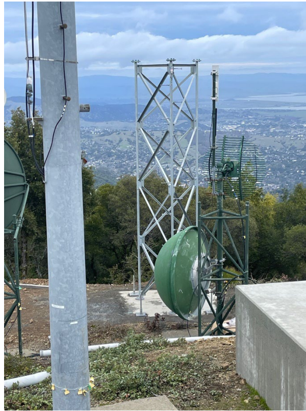
New Stub Tower
