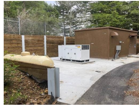
Mill Valley water tank site.
