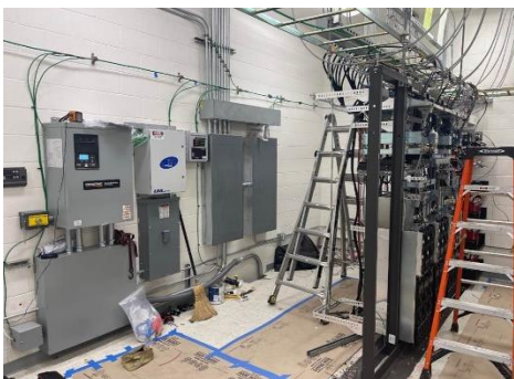
OTA Site installation in progress.
