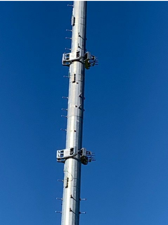
Installing Collar Mounts for the MW at Tomales
