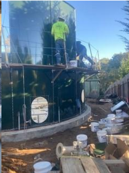
Tank #1 Wall Construction facing South
