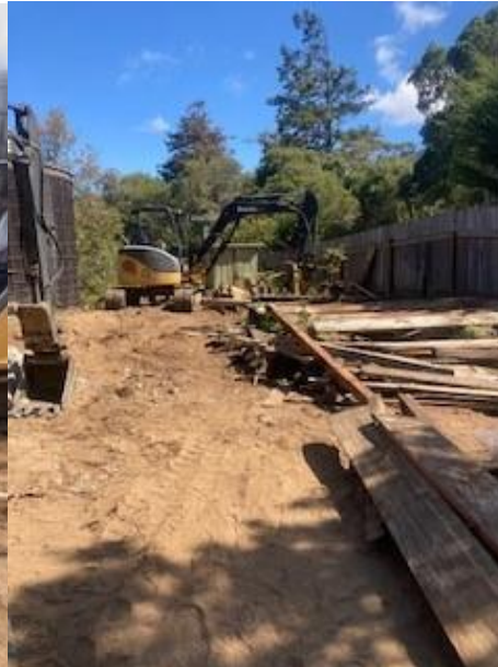
Clearing site of old tank #1, South
