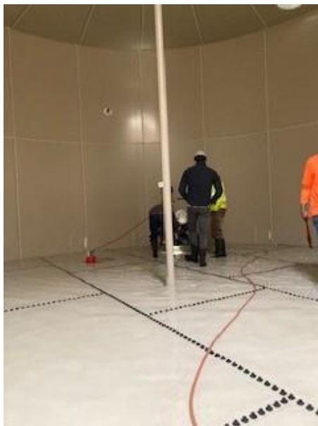
Tank #1 Interior floor vacuum test
