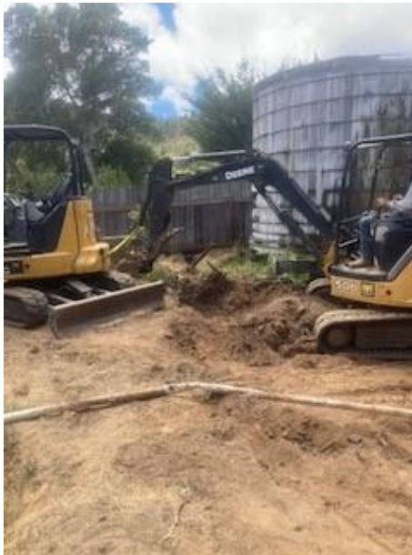
Start of project, removal of 1 st tank, South
