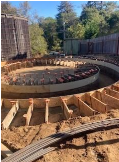
Tank #1 footing forms, facing South
