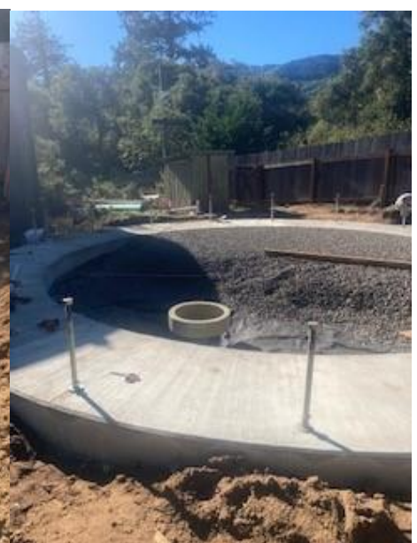
Tank #1 footing with rock underlayment
