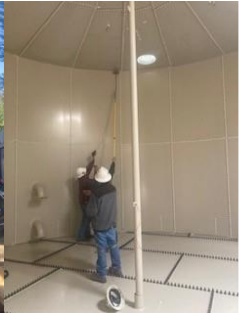
Tank #1 Interior Holiday Testing
