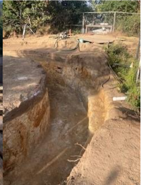
Footing for Tank #1, looking N.East
