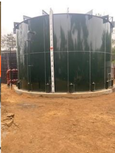
Tank #1 complete looking South
