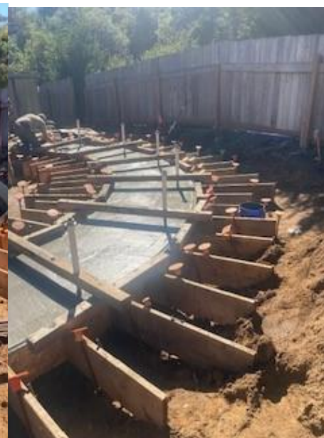
Tank #1 Footing poured, South
