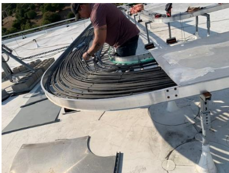
Installing Microwave cabling at the EOF site.
