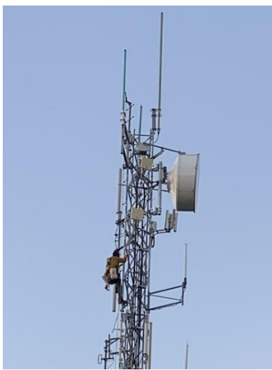
Microwave work at the Dollar Hill Site
