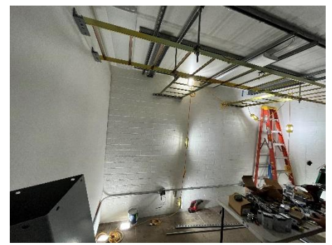
Completing electrical within the shelter at Wolfback Ridge site.
