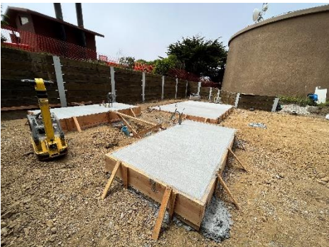
Laying foundations at Muir Beach site.
