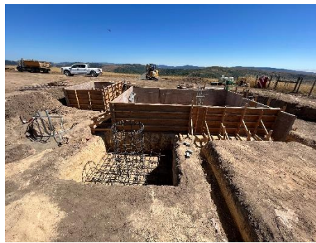
Shelter development and monopole base progress at Coyote Peak site.
