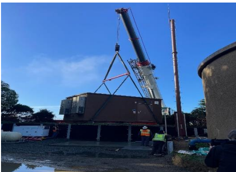
Muir Beach shelter being lifted into place.
