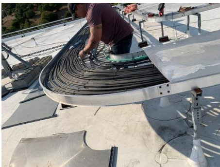
Installing Microwave cabling at the EOF site.
