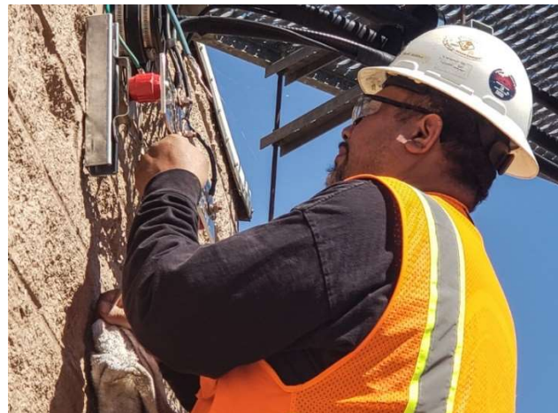
Fidato crew installing ground plate at Mr. Barnabe
