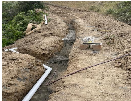
Adding drainage and backfilling the power trench at Coyote Peak.
